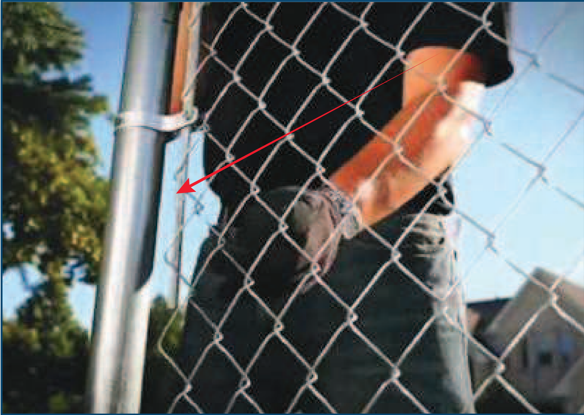
Tension bar attaches chain link panel
