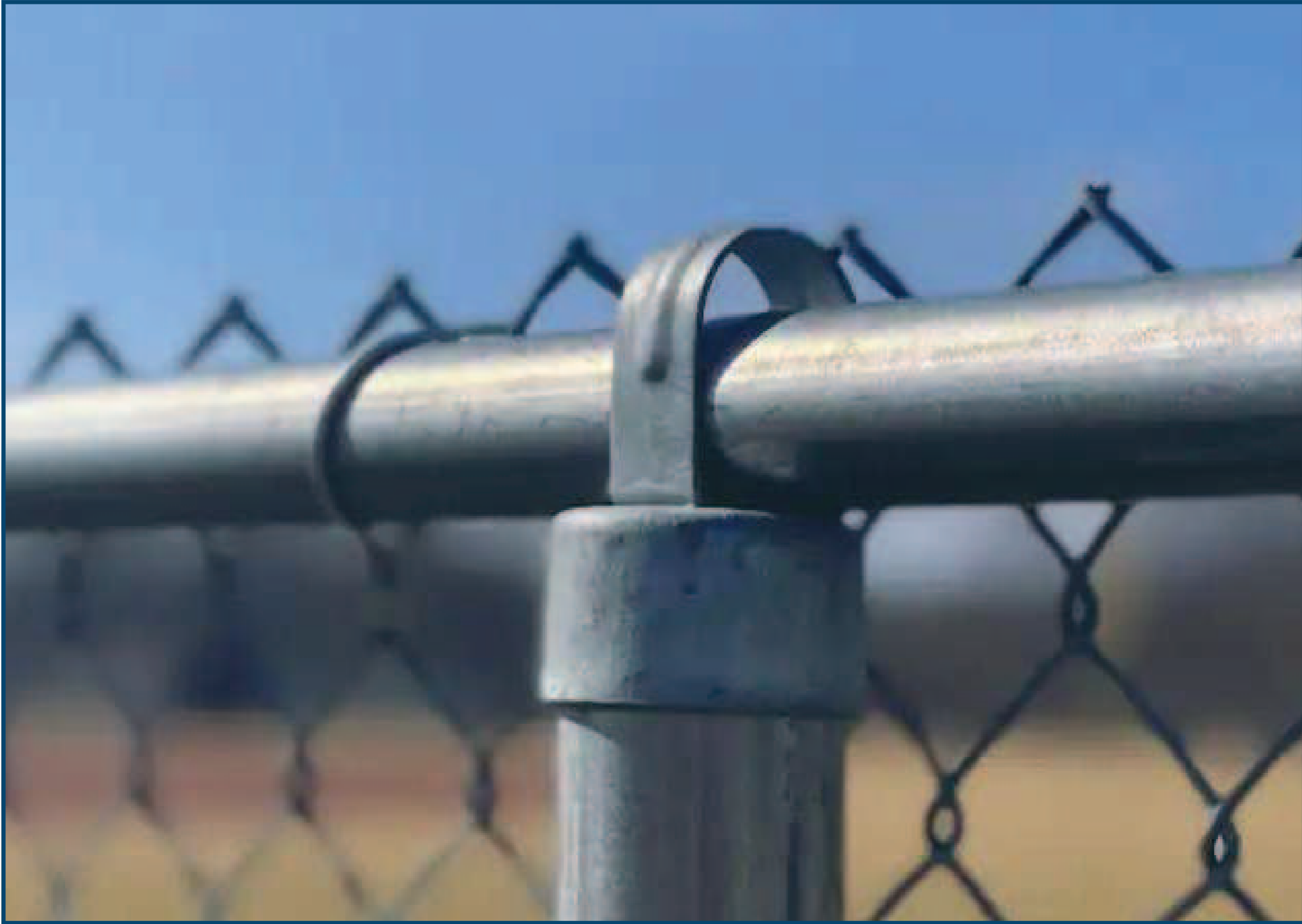
Top rail is usually at the top of fence
