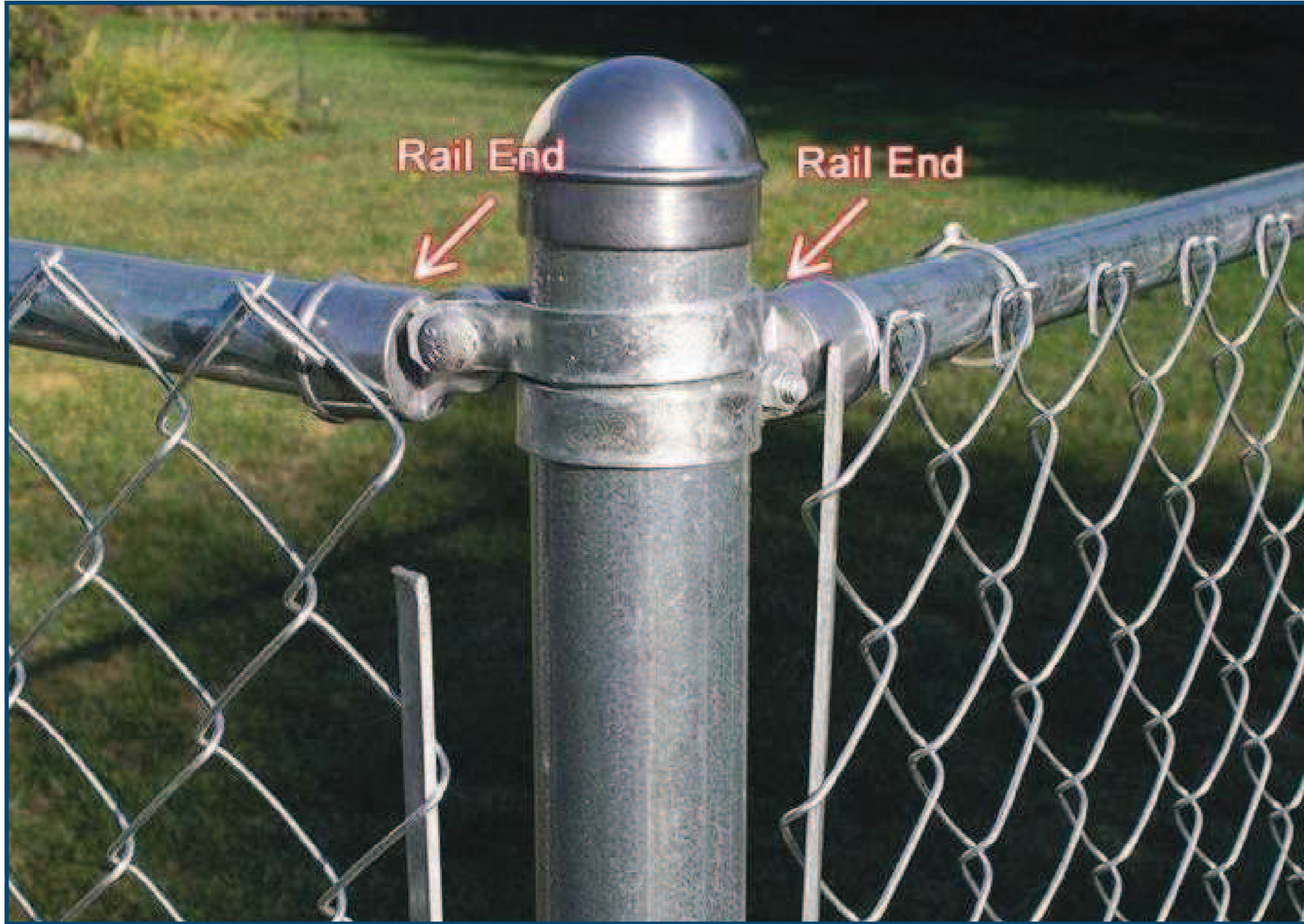
Rail end fix the horizontal post
