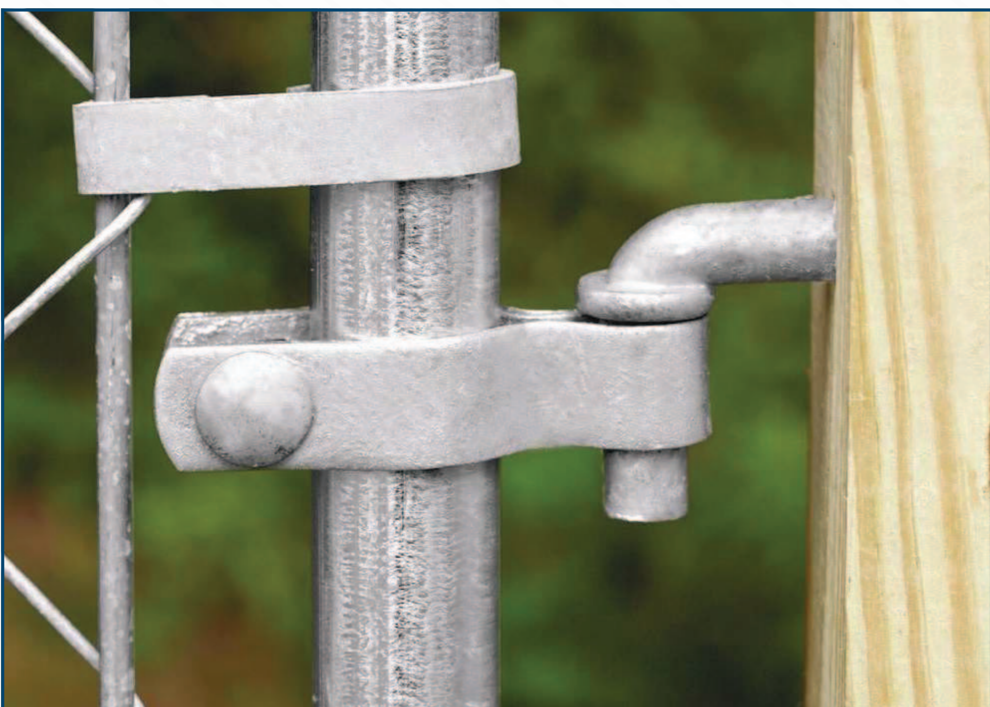
J-bolt hinge connects post to the wall
