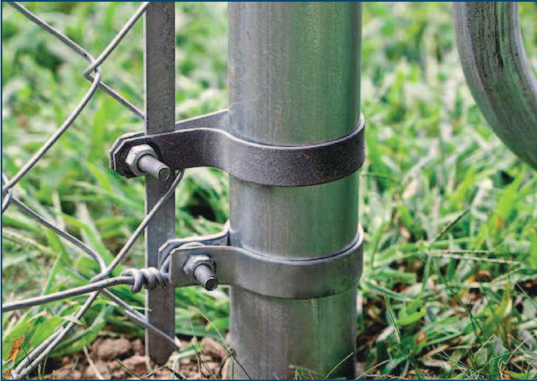
Carriage bolt tighten tension band
